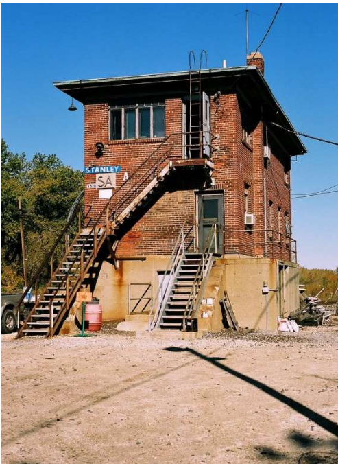
Stanley Tower, Walbridge OH just south of Toledo, demolished in 2017. J Thompson Jr. photo, 1969 https://wd8rif.com/img/jt3.jpg
